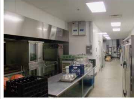
View of Banquet Kitchen Area
