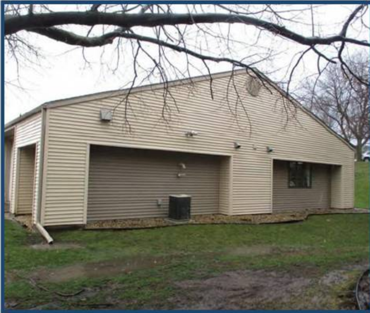
North Elevation of Building Facing South
