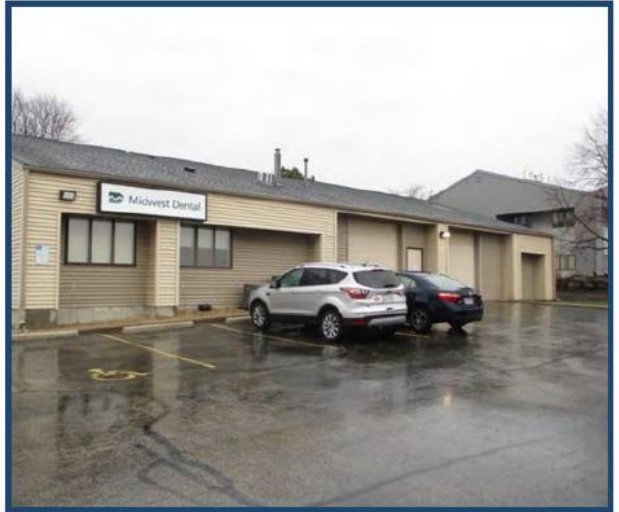
East Elevation of Building Facing West
