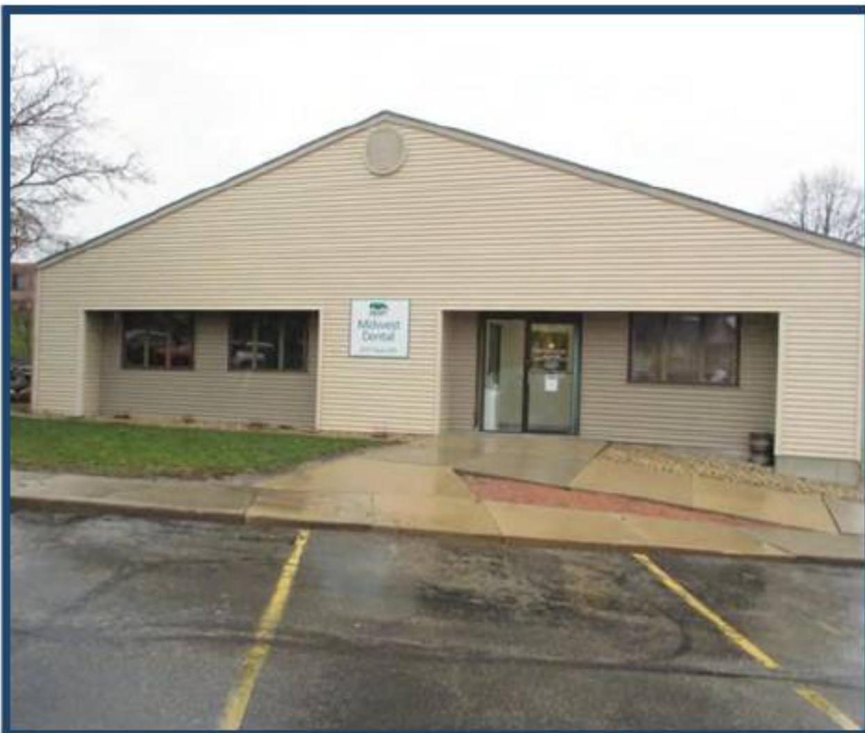
South Elevation of Building Facing North
