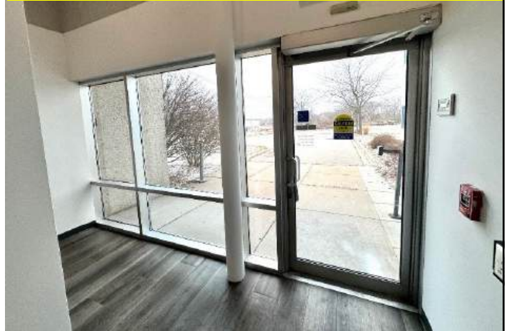
Back Parking Lot Entrance
