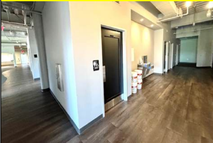
Restrooms/ Elevator Access
