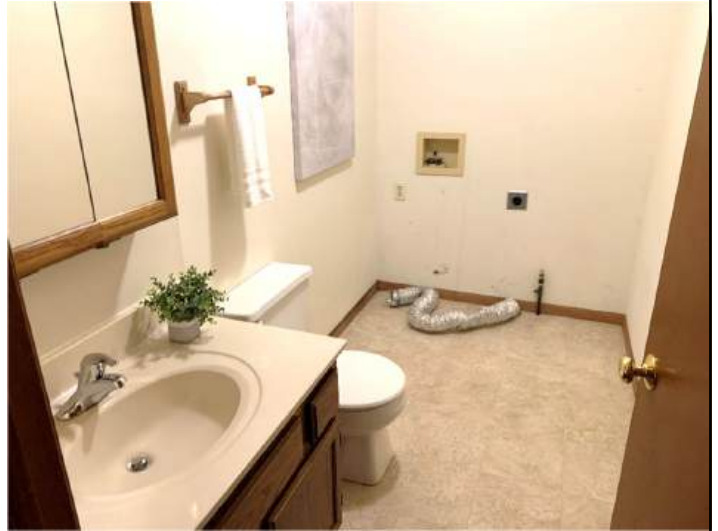
Washer/Dryer Hook Ups
