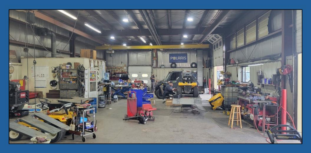
Building #3 is located to the south of the Main Building. This building serves as shop space and has interior and exterior walls that are about 50 percent concrete block and 50 percent metal, with concrete flooring and exposed ceilings. The pitched metal roof is about 16 feet high at the eaves. This building is divided into two rooms. There are 3 overhead doors and one overhead crane. Total building size is 6,400 square feet. Heat is provided by gas-fired, ceiling mounted radiant tubes.
