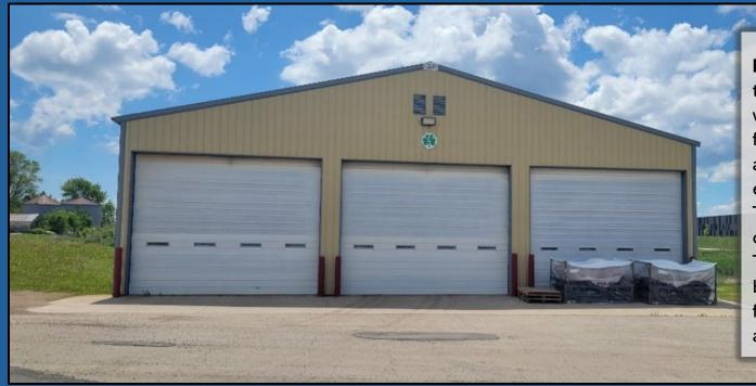
Building # 4 is located a short distance to the west of the Building #3. It is a wood-framed pole type structure used for storage. The space is comprised of a single open area. The building has electrical service but is unheated. There is metal panel exterior siding over a wood frame with gravel flooring. There are 3 overhead doors in this building. Building size is 4,200 square feet. The building is about 16 feet high at the eaves.
