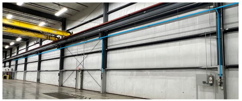
16 compressor distribution points throughout the building. Includes Kaeser Rotary Screw ASD 40 Compressor. 40 hp, 91 CFM capacity, 125 psig operating pressure range, with Ingersoll Rand Refrigerator Air Dryer.
